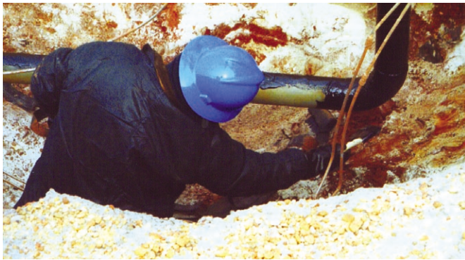
Brush application of coal tar coating.
