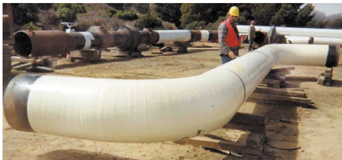
(Right) Rubberized bitumen tape applied to steel pipe.
