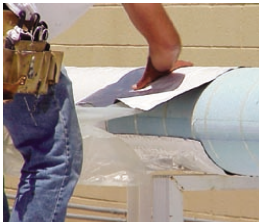
Application of rubberized bitumen vapor retarder/weather barrier membrane on ammonia refrigeration piping system.
